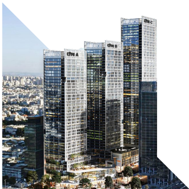
LYFE, Building C, Bnei Berak Building rights (100%): ~90,000 m 2 Ownership: 50%
