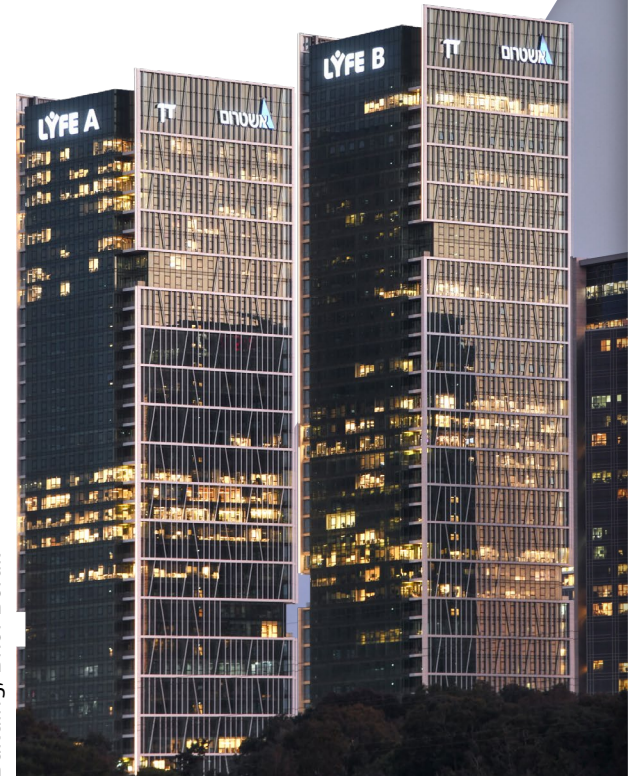
LYFE, Building, Bnei Berak
